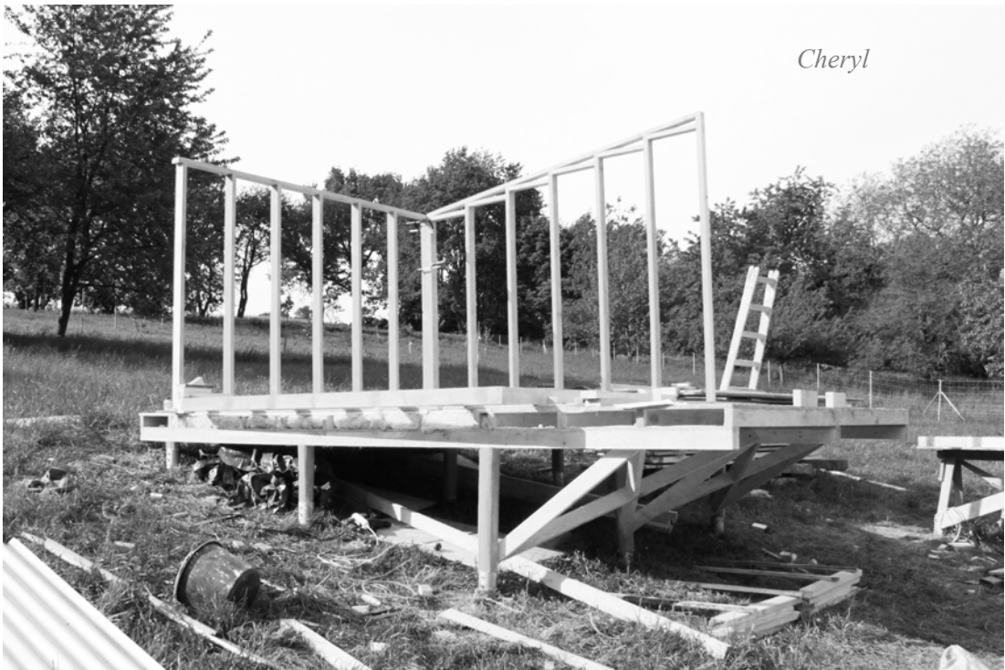
Erecting the first two wall frames
