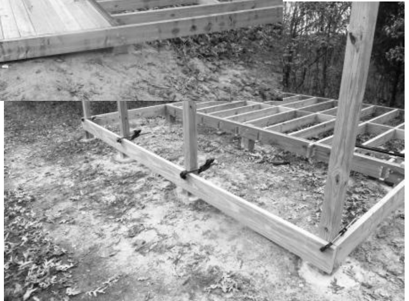
Floor framing - cabin Bettie; Texas
