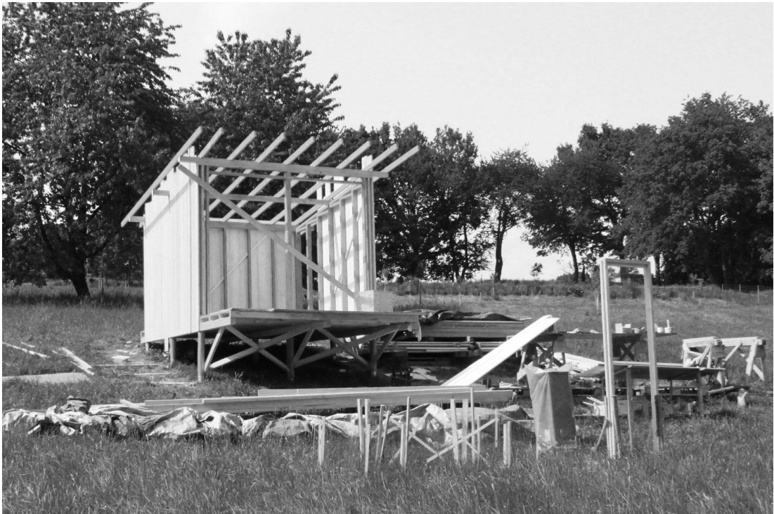
Constructing the trusses, Cheryl, Czech Republic
