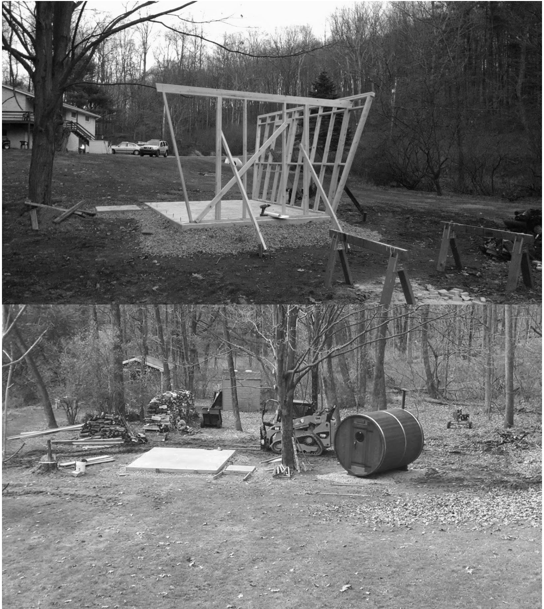
Foundation slab - Ann; East Pennsylvania
